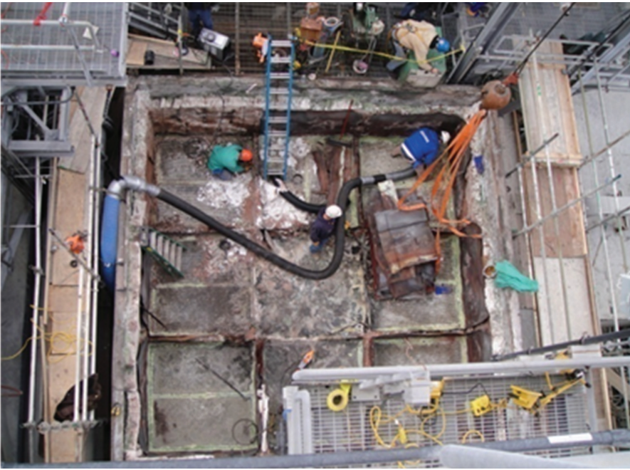
The old ceramic media is removed from the heat-recovery baskets.
