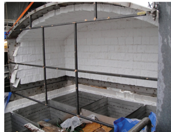
The heat-recovery baskets were rebuilt and reloaded with new media.
